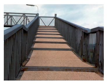
Preformed Surface Dressing is an exceptionally versatile, ready-to use, hard wearing skid resistant surface for pedestrian trafficked areas. Preformed Surfacing Dressing comprises a high performance polymer modified bituminous binder and a layer of skid resistant calcined bauxite chippings strengthened by an integral mesh. Preformed Surface Dressing can be used on most surfaces, including wood, concrete, asphalt and steel.
